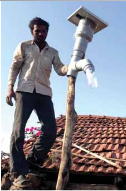
A solar lighting system being erected in a rural home.
